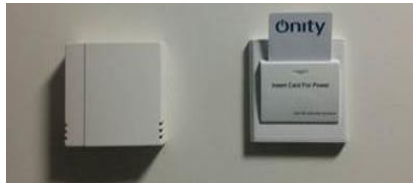
Example of thermostat and card on/off switch, with air conditioning set to 'on'.
