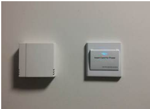
Example of thermostat and card on/off switch, with air conditioning set to 'off'. The blue light activates once the ducting has closed.
