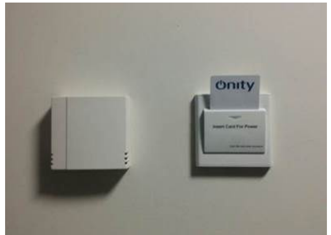
Example of thermostat and card on/off switch, with air conditioning set to 'on'.
