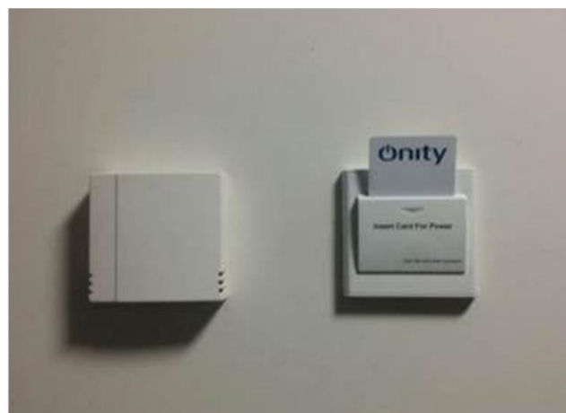
Example of thermostat and card on/off switch, with air conditioning set to 'on'.
